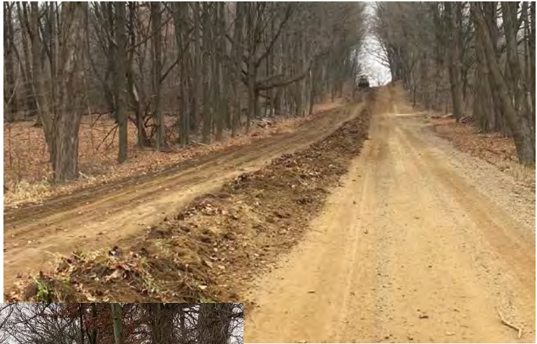
Prep work to remove debris and organic shoulder material in progress (above) and completed (left).
