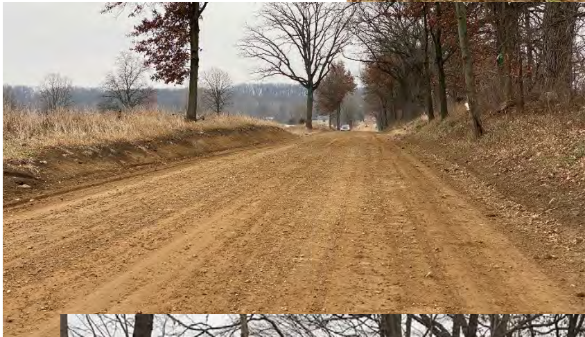
Prep work to remove debris and organic shoulder material in progress (above) and completed (left).
